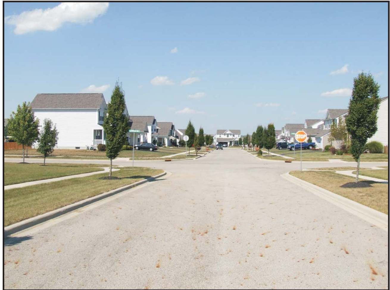
Figure 27: A residential subdivision within Etna Township.
