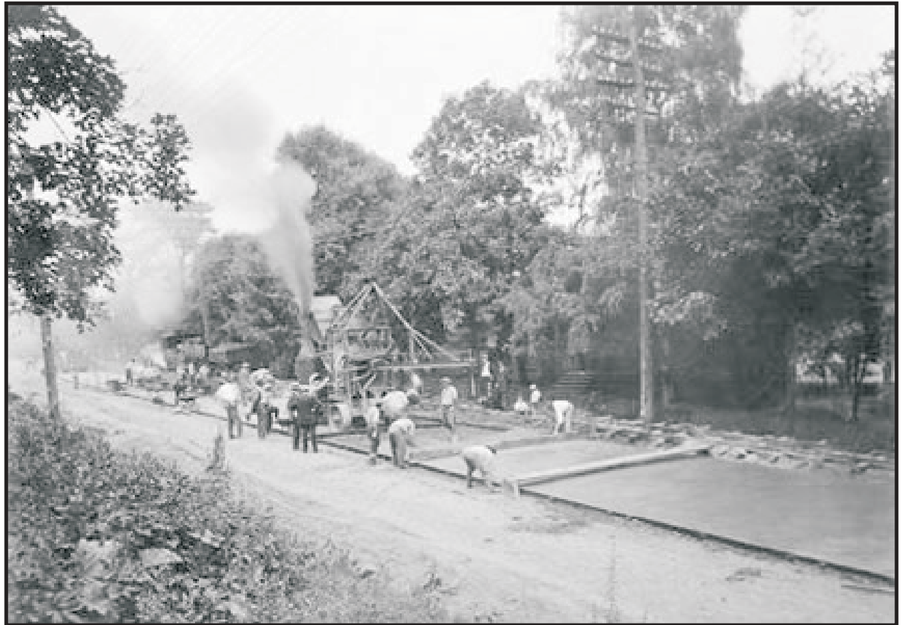
Figure 4: The construction of US 40 through Etna Township.
