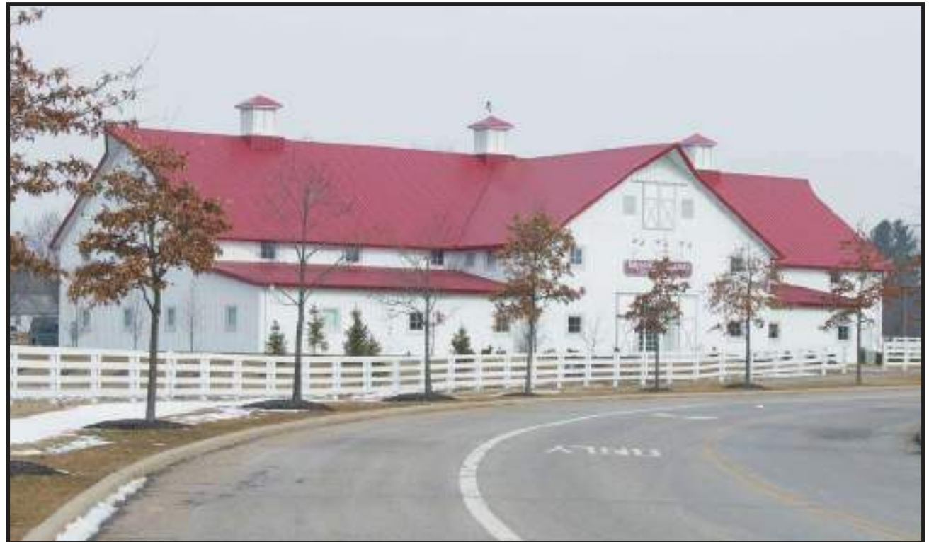
Figure 62: Commercial developments should incorporate rural design elements.
