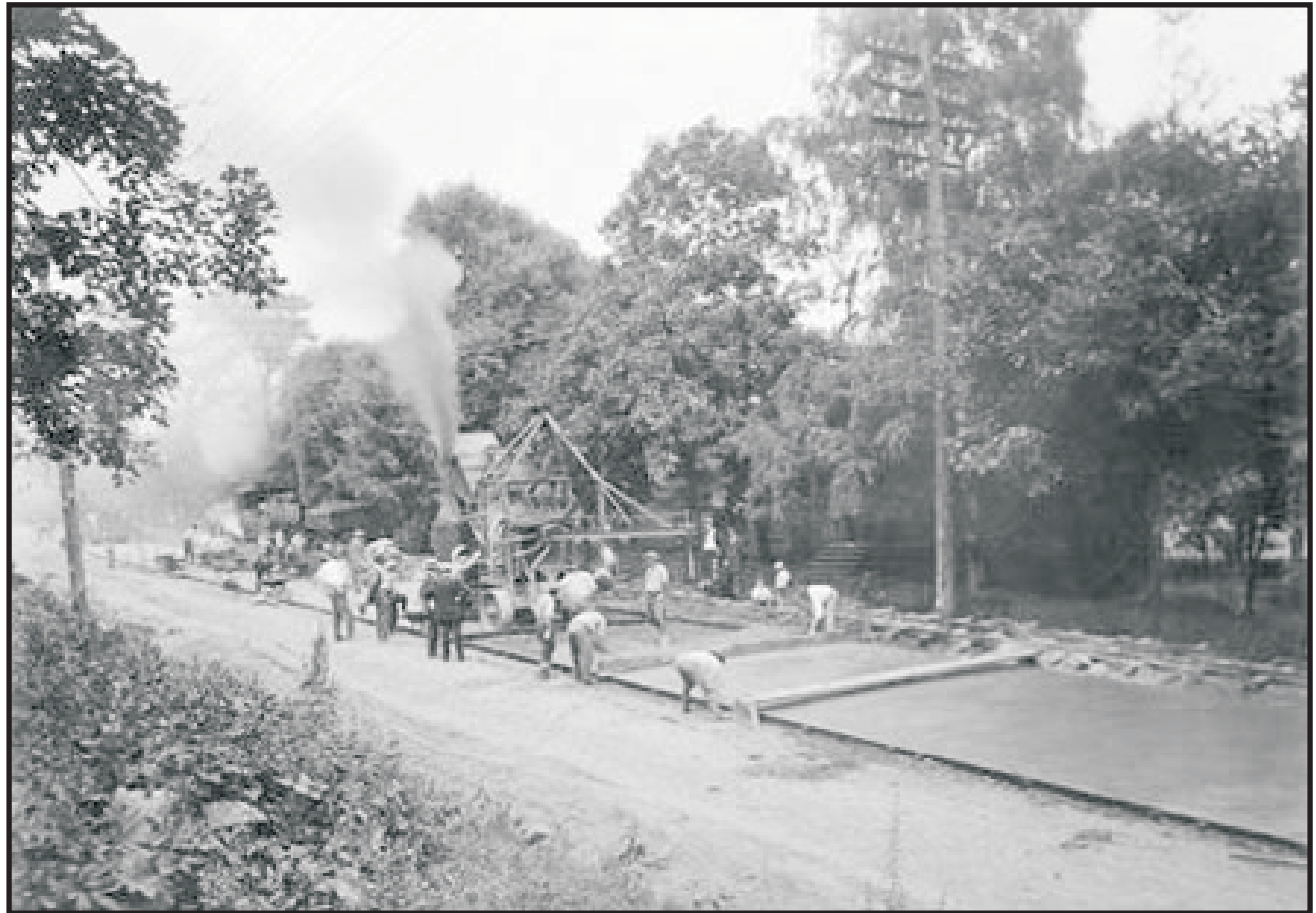
Figure 4: The construction of US 40 through Etna Township.
